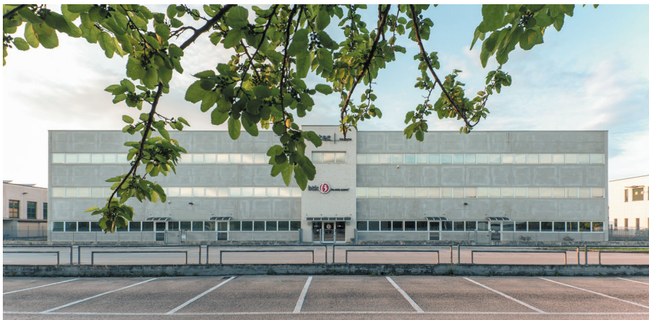
BTK Headquarters - NORTH ITALY
